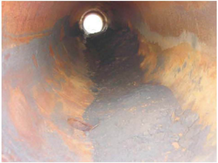
Figure 5. Iron oxide sediment in a 508 mm pipeline. The volume of sediment can be enormous and should be considered in pig cleaning operations.
